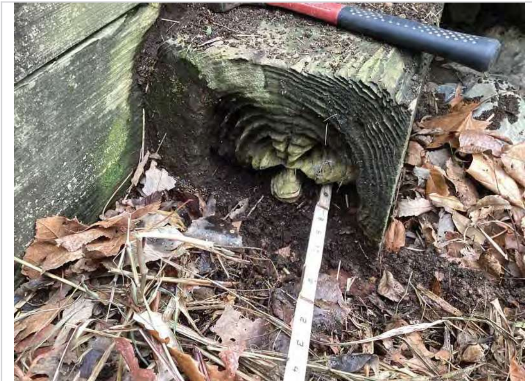
Abutment 2 cap left end decayed area
