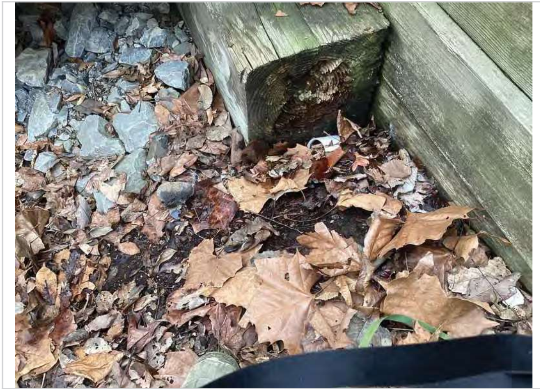
Abutment 2 right end cap decayed area
