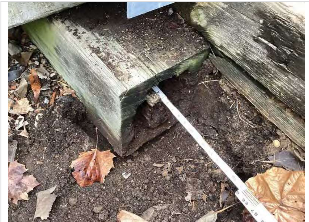
Abutment 1 left side of cap decay
