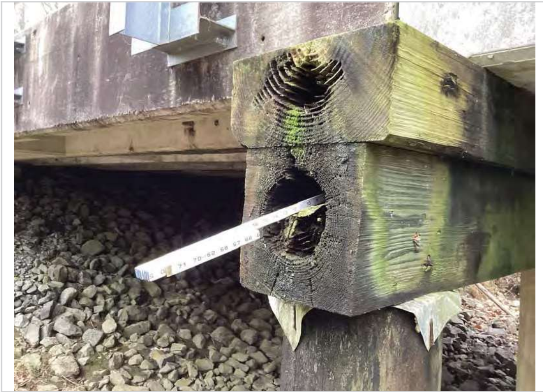
Bent 1 left side of cap "B" decay
