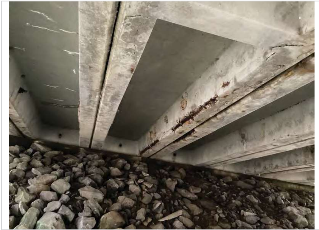
Span 2 precast concrete slab "D" spall to steel
