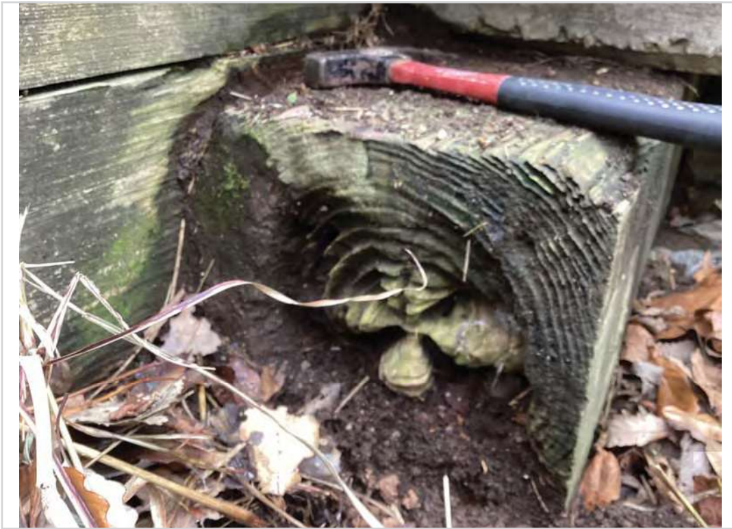
Abutment 2 cap left end decayed area
