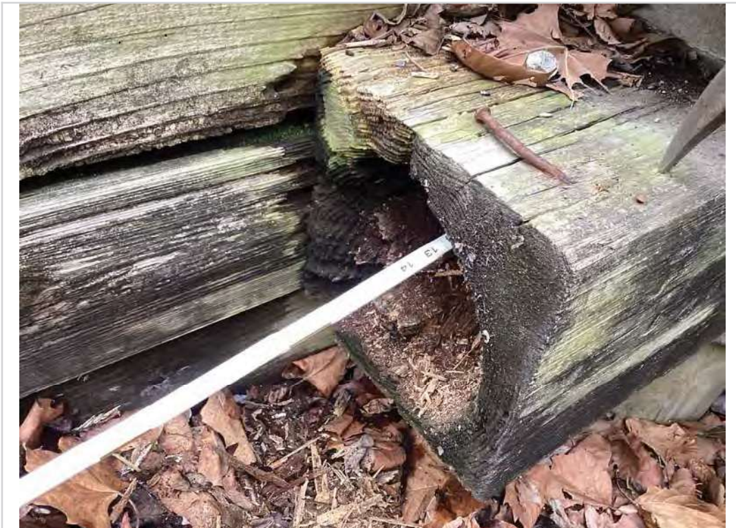
Abutment 1 right side of cap decay
