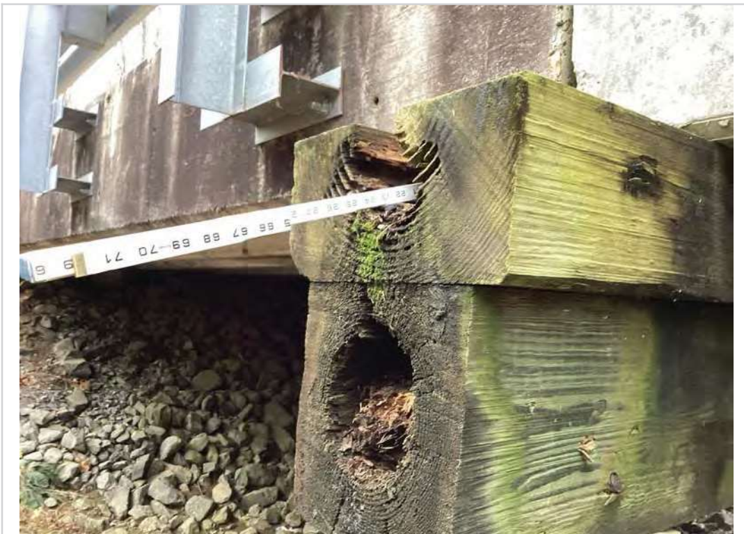
Bent 1 left side of cap "A" decay
