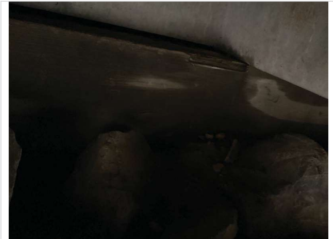
Abutment 2 cap splintered area. Medium weathering
