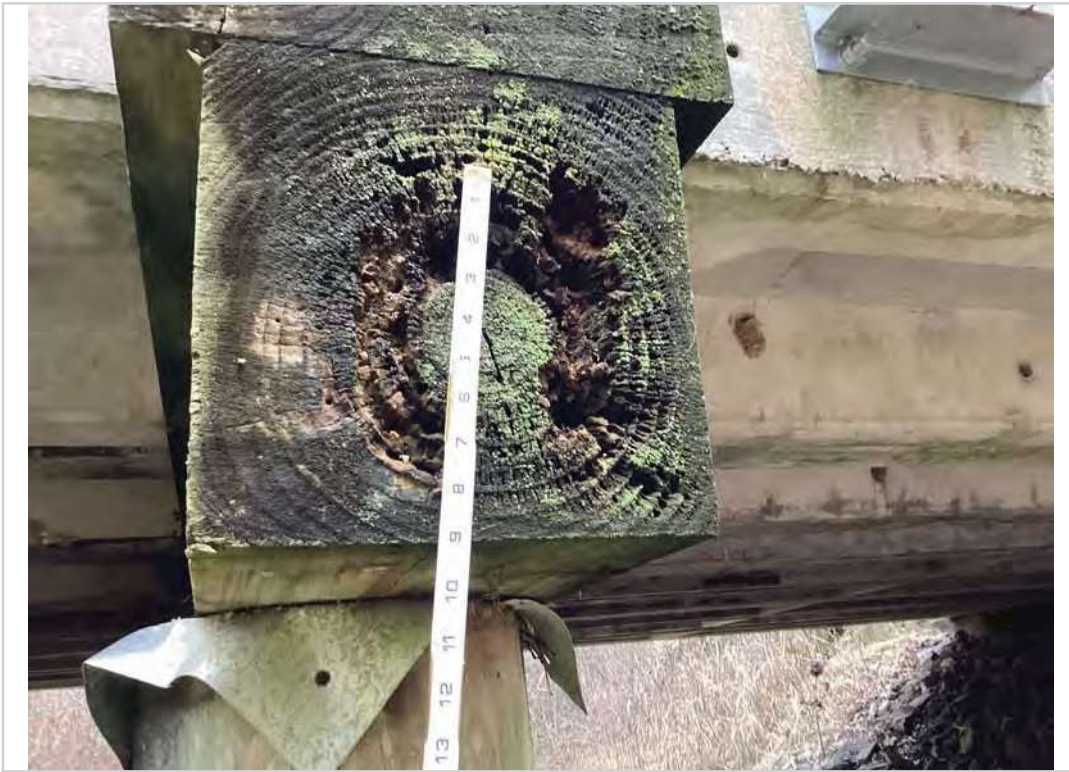
Bent 1 right side of cap "B" decay
